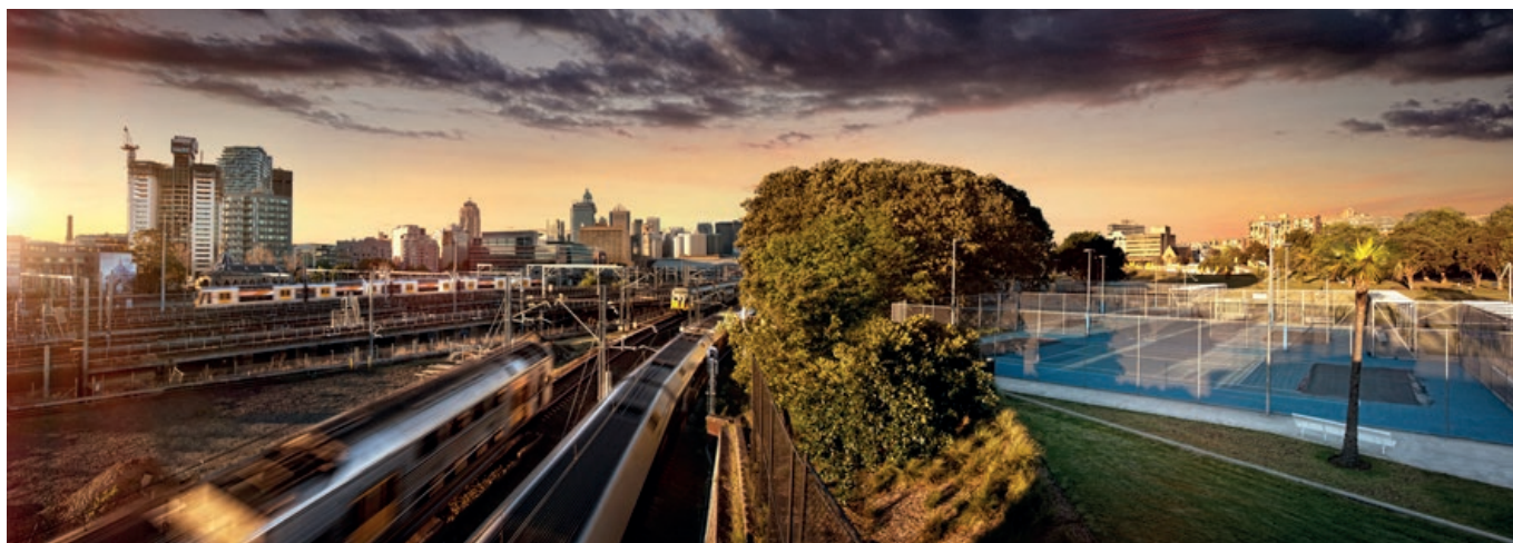
City infrastructure: rail lines, shade trees and tennis courts, Prince Alfred Park, Surry Hills. Photo: Joseph Nalevansky.
